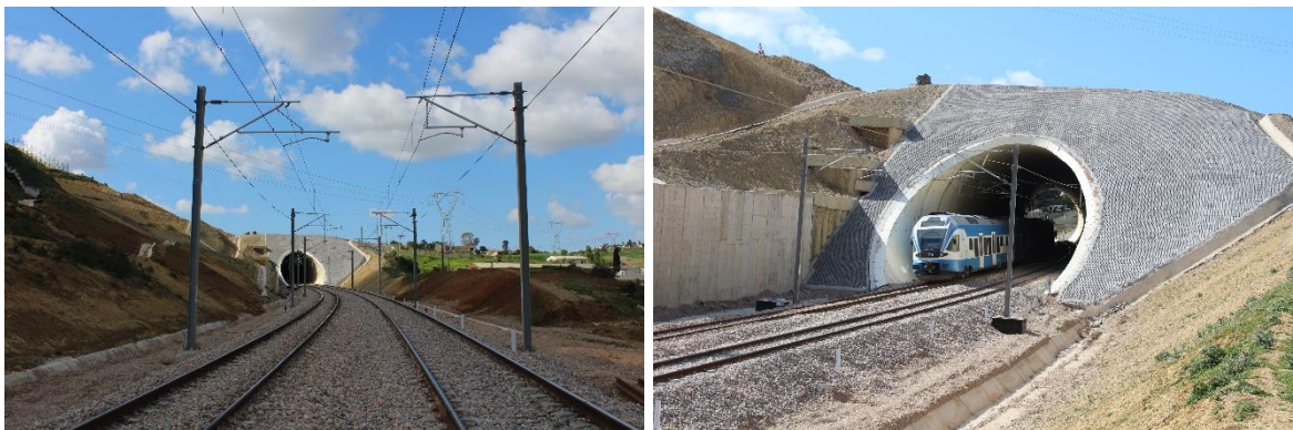
Figure 18. Tunnel en service
